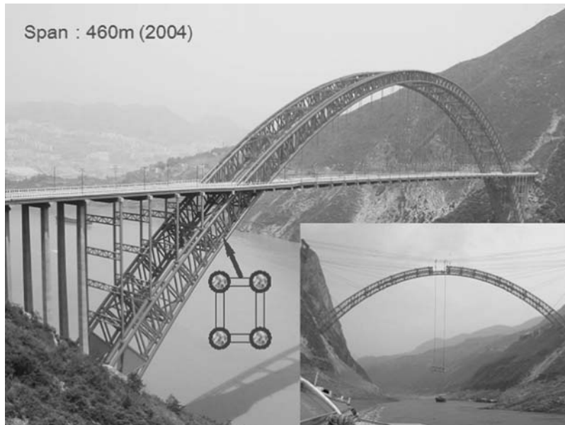
Figure 6-55 Wushan CFST arch bridge, Chongqing China
