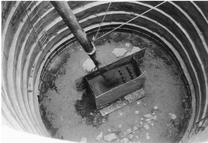
Figure 3-21 Drop chute-guided concrete fall
