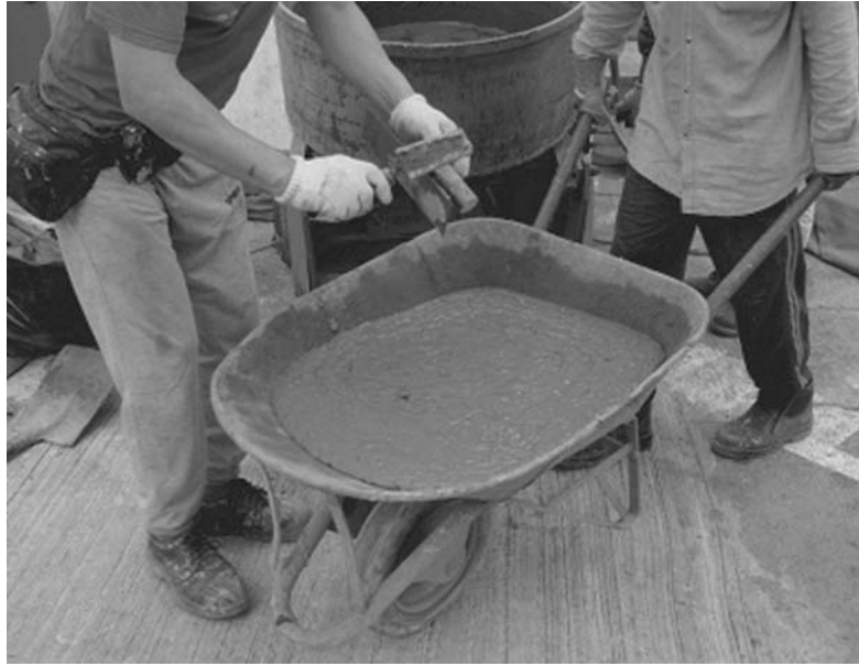
Figure 3-19 Wheelbarrow used on construction site
